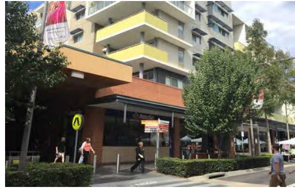
Photo 6.4. Major building entries need to be clearly identified and connected to the pedestrian network.
